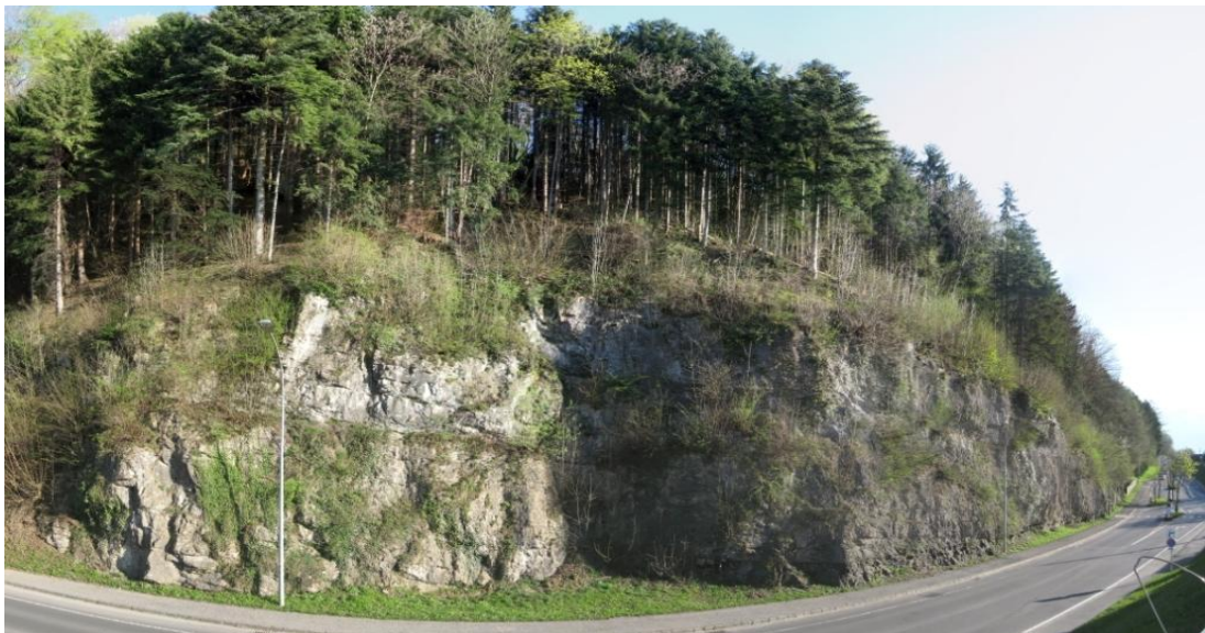
Tunnel portal area Tosters (north-eastern project area)
